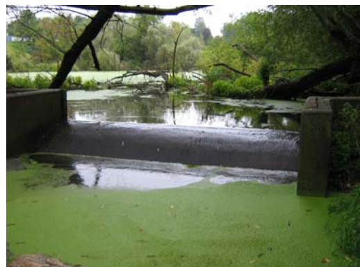
A Low-Head Dam Fragmenting Aquatic Habitats in an Ozaukee County Creek
